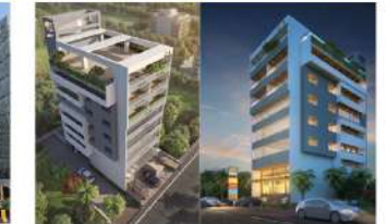
• NIRMAN BHARATHI CITY CENTER- A+T BUILDING, AURANGABAD
